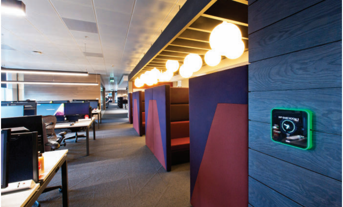
FIG. 3. Tunable lighting at the Registers of Scotland offices is managed via iPad controls from Casambi mounted on the walls.
